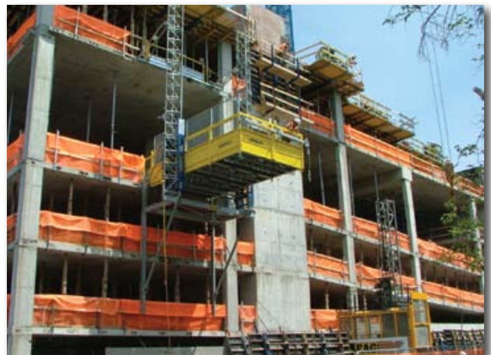
The TLS can be installed on the ground floor, allowing for an efficient cycle of tables throughout the entire project.
