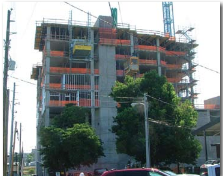
The Table Lifting System (TLS) is an electric-powered lifting platform that allows preassembled tables to be cycled between floors on a building structure without the need for a crane. It takes the crane requirement completely out of the formwork cycle and makes it available for other tasks.
