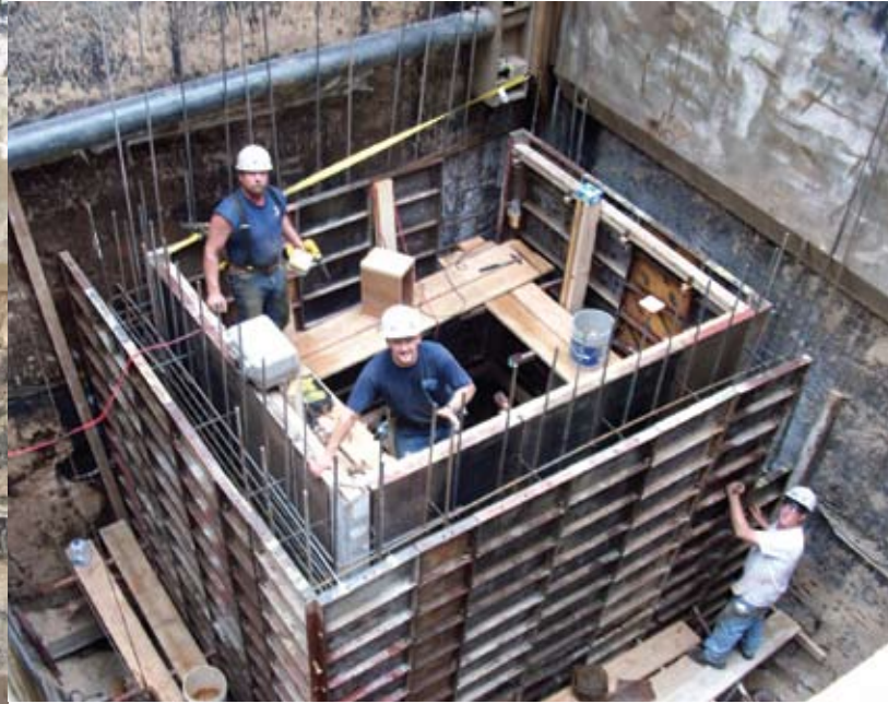
Left: McCormick Sand, Inc., excavated and shored a 28-foot-deep pit in preparation of casting-in-place a new elevator shaft. When the system was installed, the corner posts were tied back with chains so that the panels and parallel beam assembly along the building's perpendicular exterior walls and the linear post in the building's apex could be pulled up 16 feet to make room for the elevator shaft.
