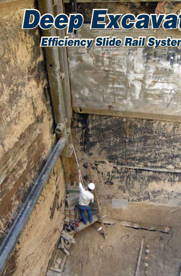
Left: McCormick Sand, Inc., excavated and shored a 28-foot-deep pit in preparation of casting-in-place a new elevator shaft. When the system was installed, the corner posts were tied back with chains so that the panels and parallel beam assembly along the building's perpendicular exterior walls and the linear post in the building's apex could be pulled up 16 feet to make room for the elevator shaft.
