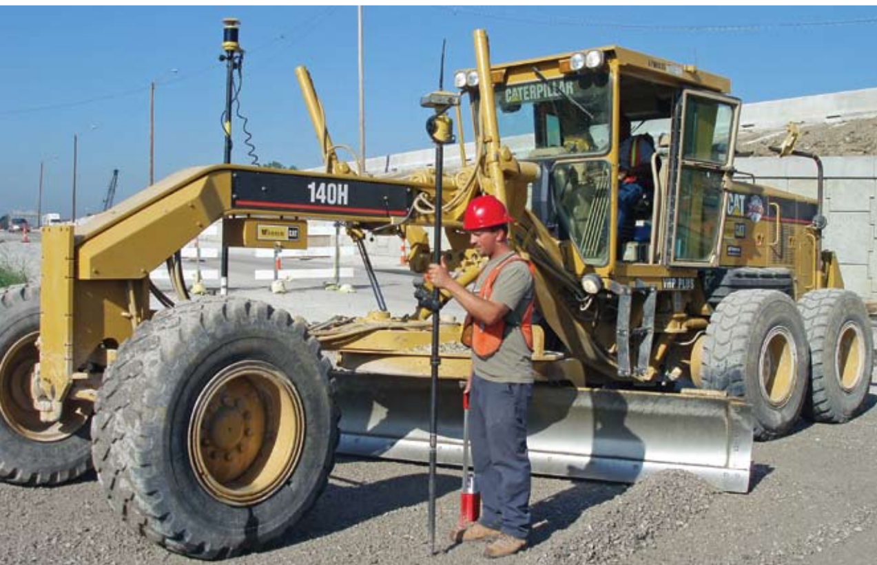
Above: Larry Cox of Heber Springs, Arkansas, grade checks in front of a machine-controlled grader.
