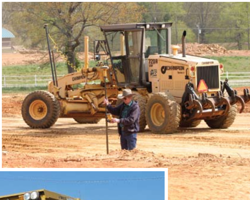
Above: Larry Cox of Heber Springs, Arkansas, grade checks in front of a machine-controlled grader.
